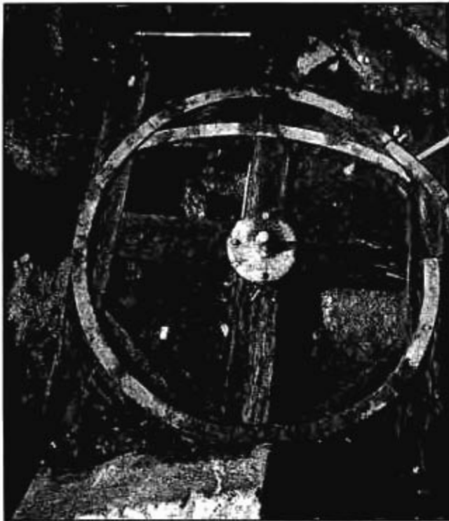
Figure 15.7. (left) Near-overhead Rolleimetric perspective image of an exposed iron and wood cannon-testing platform discovered at West Point Foundry.
