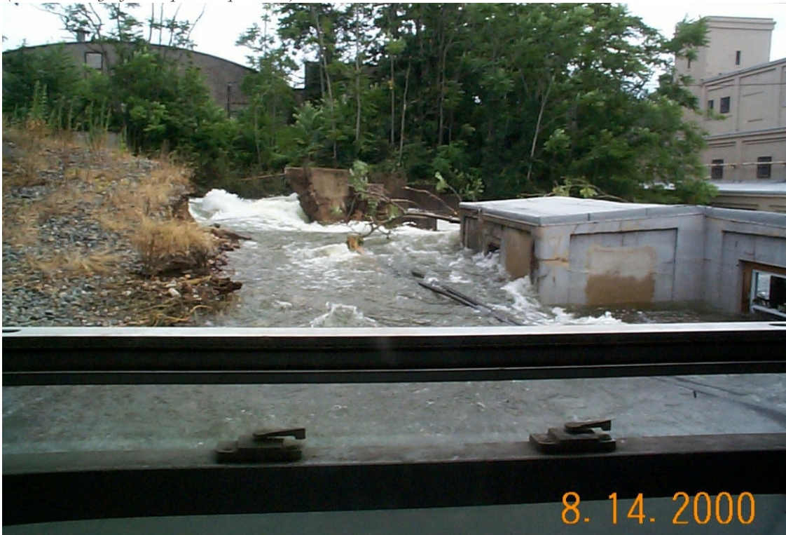
Figure 21. Field shot looking due south at Lower Spillway documenting extent and depth of scour erosion during August 2000 dam breach and flood at the Compact Corporation site in Stanhope/Netcong, New Jersey (Photo courtesy of Compac Corporation ).
