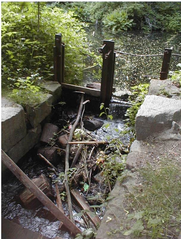
Figure 10. Contemporary field views of “Foot” of 1840’s L-shaped Spur, or “ Raceway to the Works ”, above the Foundry, looking south in the direction of Furnace Pond ( Top ); Detail looking north, towards south bank of the L-Shaped Spur, at mid-19th century cut stone and iron Sluice Gate, which regulated water discharge to both the Foundry and Furnace Pond below ( Bottom ) (Photos by Joel W. Grossman, Ph.D., June 23, 2002).
