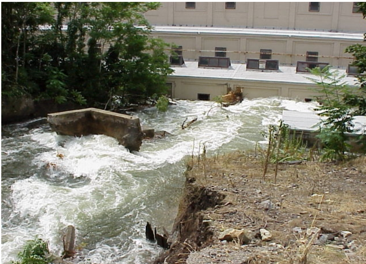
Figure 22. Field shot looking west, downstream, at Lower Spillway showing north-south extent and depth of scour erosion during 2000 Musconetcong flood at the Compact Corporation site in Stanhope/Netcong, New Jersey ( Photo courtesy of NJDEP ).
