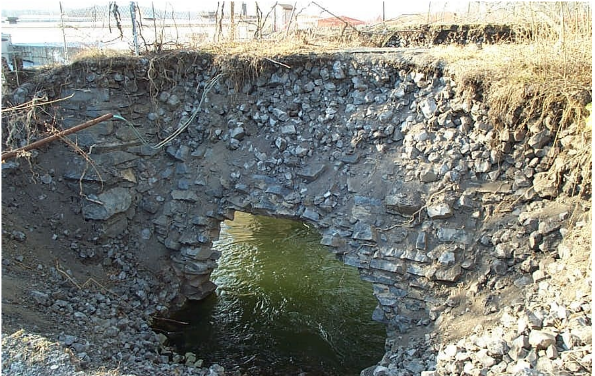
Figure 28. View looking north-west at deep erosion induced collapse of southern half of earth filled and cut stone clad 1874 arched bridge at Furnace Pond Dam( Photo courtesy of NJDEP )
