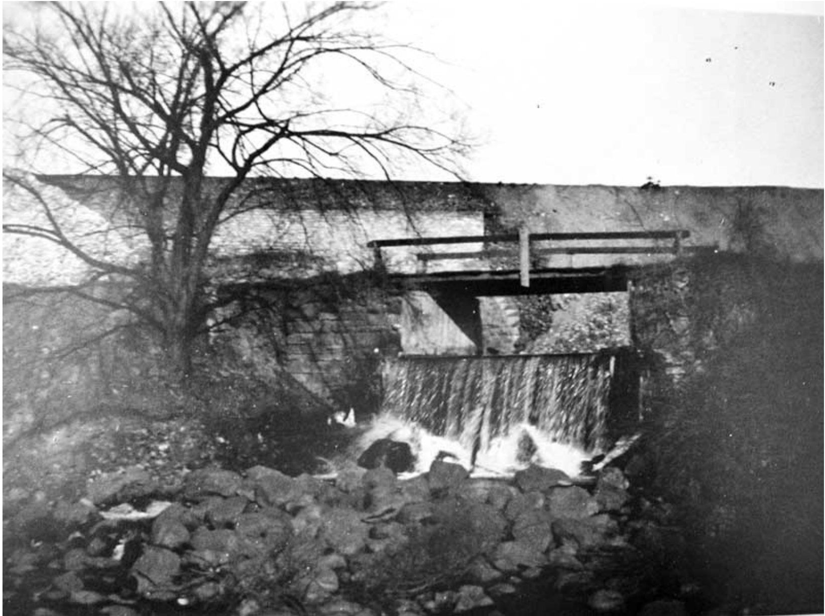
Figure 13. Undated (pre 1927) historic photograph of the “Singer Lower Spillway” showing 19th century motored stone abutment and wing wall supporting former footbridge ( Photo courtesy of Musconetcong Foundrymen Historical Society )
