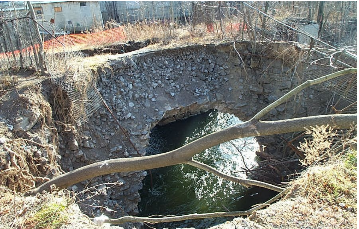
Figure 28. View looking north-west at deep erosion induced collapse of northern half of earth filled and cut stone clad 1874 arched bridge at Furnace Pond Dam( Photo courtesy of NJDEP )
