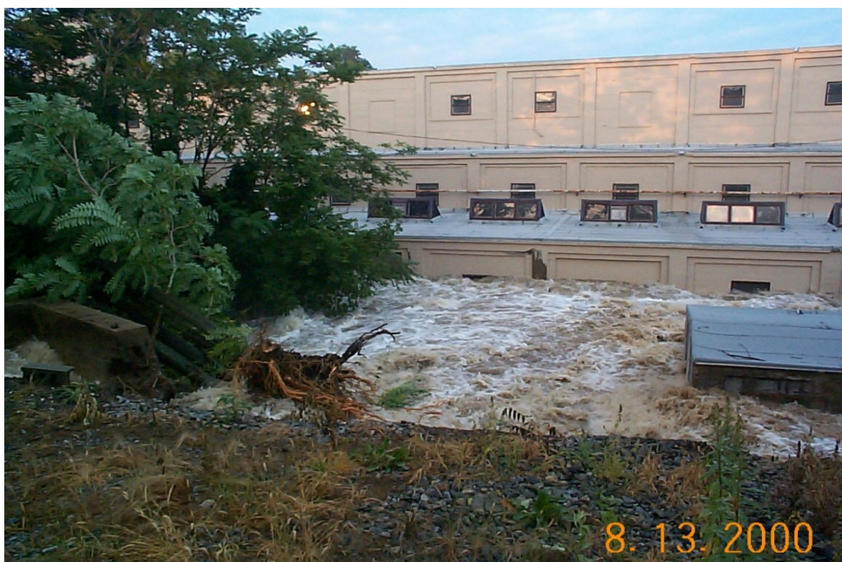
Figure 23. Field shot looking west, downstream, at Lower Spillway showing depth of scour erosion in Stanhope/Netcong, New Jersey ( Photo courtesy of Compac Corporation ).
