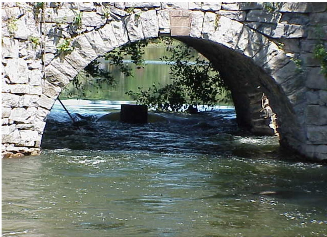
Figure 24. Field shot looking east, upstream, through arch of cut stone bridge showing collapsed earth filled core on right interior at the Compact Corporation site in Stanhope/Netcong, New Jersey ( Photo courtesy of NJDEP ).
