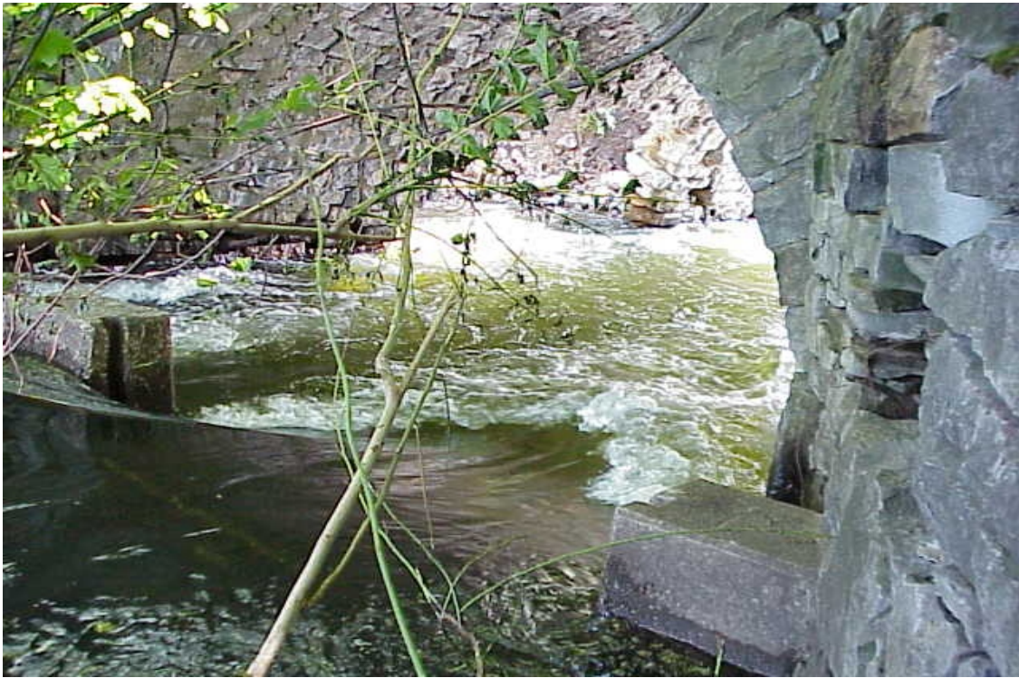
Figure 26. View looking south, across 1927 cement weir pods, into interior arch of former cut stone bridge at Furnace Pond showing partial collapse from flooding of central core of earth filled structure ( Photo courtesy of NJDEP ).
