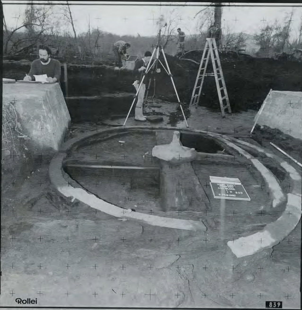
View of excavated gun-testing platform taken with ultra-high-resolution 3-d photogrammetric camera for plotting on computer mapping system. GROSSMAN AND ASSOCIATES
